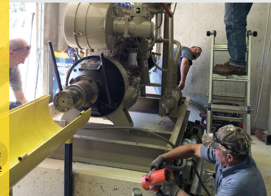
Toquerville new engine installation
