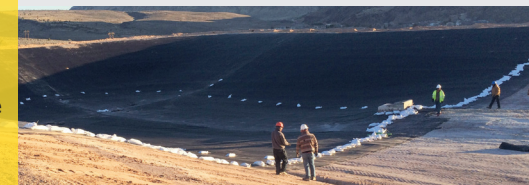
Toquerville pond liner install
